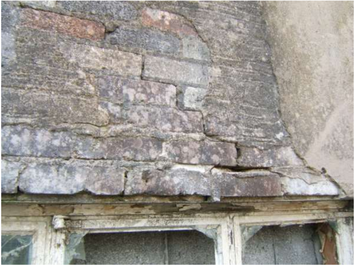
COLLAPSE OF BRICKWORK & LOSS OF BRICK BOND ABOVE R.H.S. REAR WIDE WINDOW ON GROUND FLOOR
