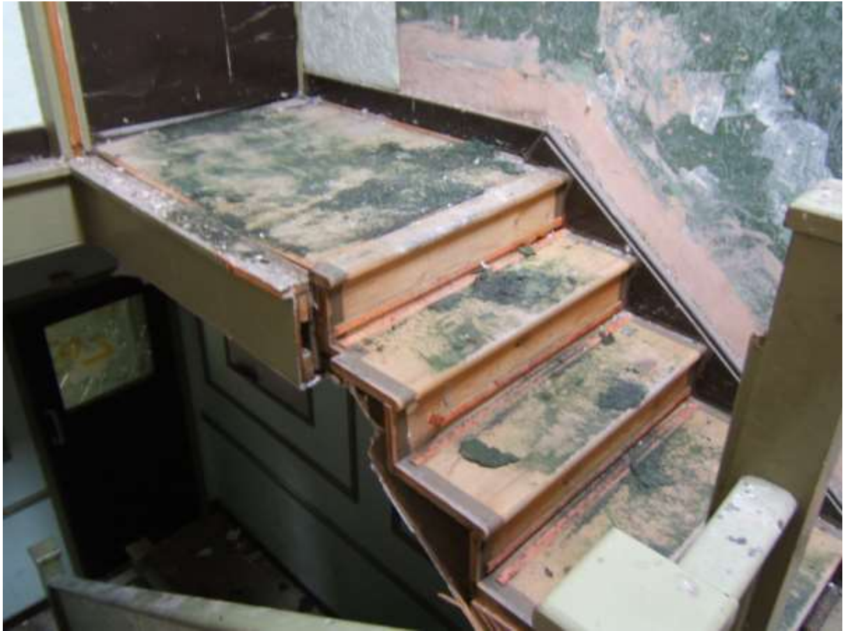
DAMAGED & UNSUPPORTED UPPER AREA OF TIMBER STAIRS
