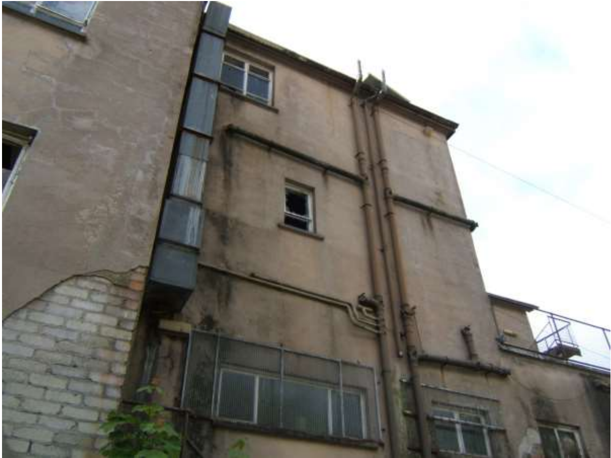
UPPER REAR ELEVATION WITH RENDER DEFECTS TO WALL
