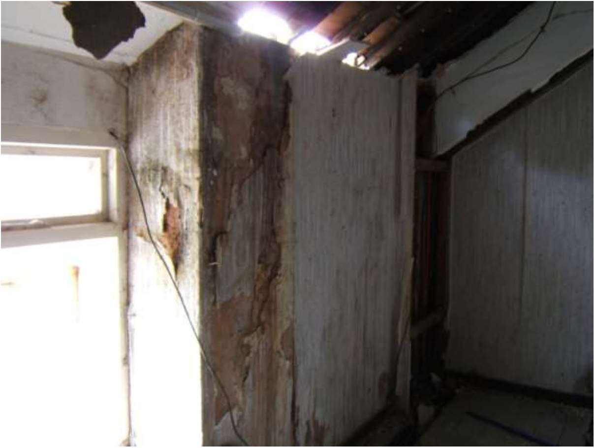
WATER DAMAGED UPPER REAR WALL INTERNALLY
