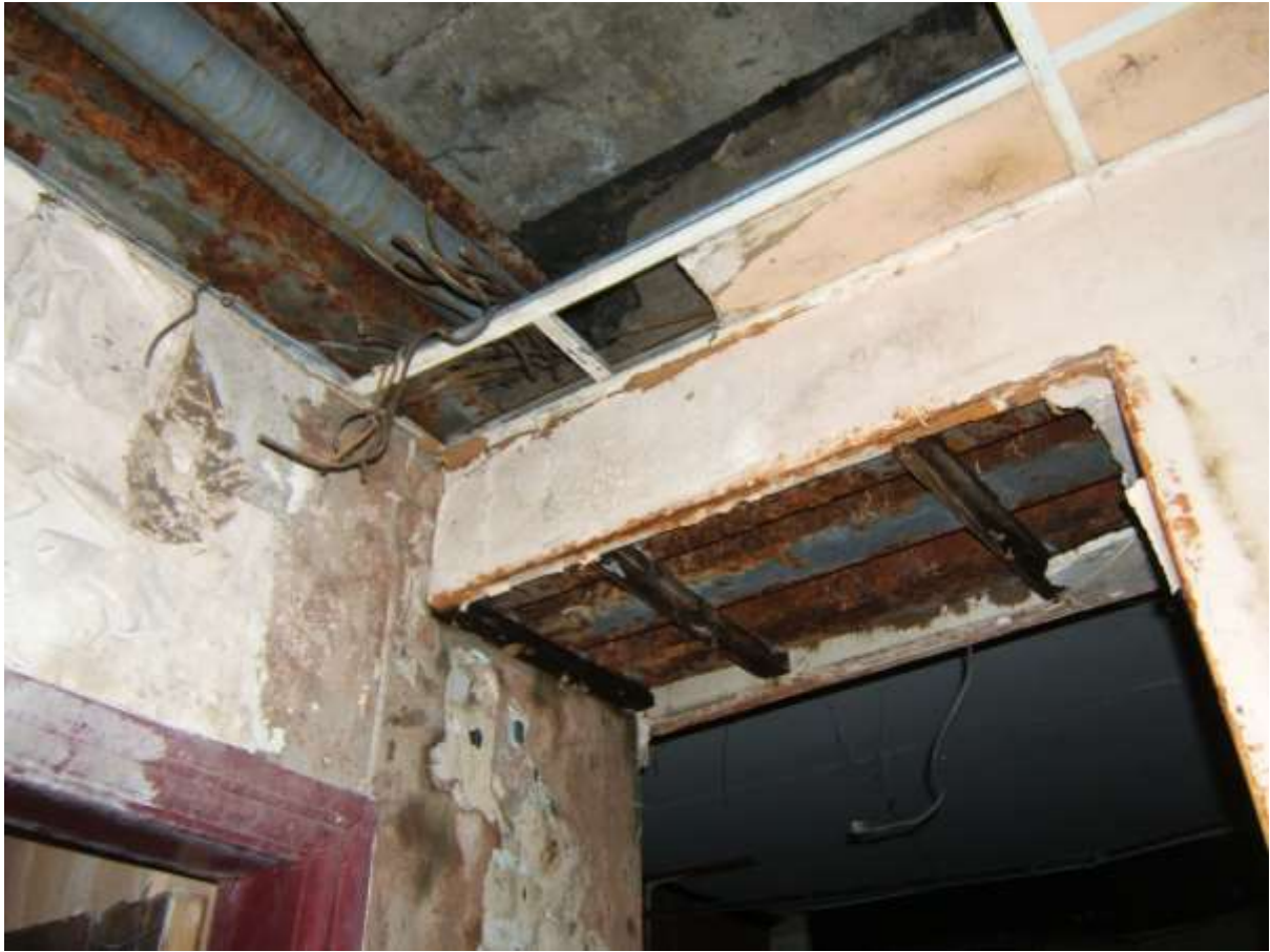
WATER DAMAGED STEEL SUPPORTING MEMBERS INTERNALLY ON GROUND FLOOR FORMER BAR AREA
