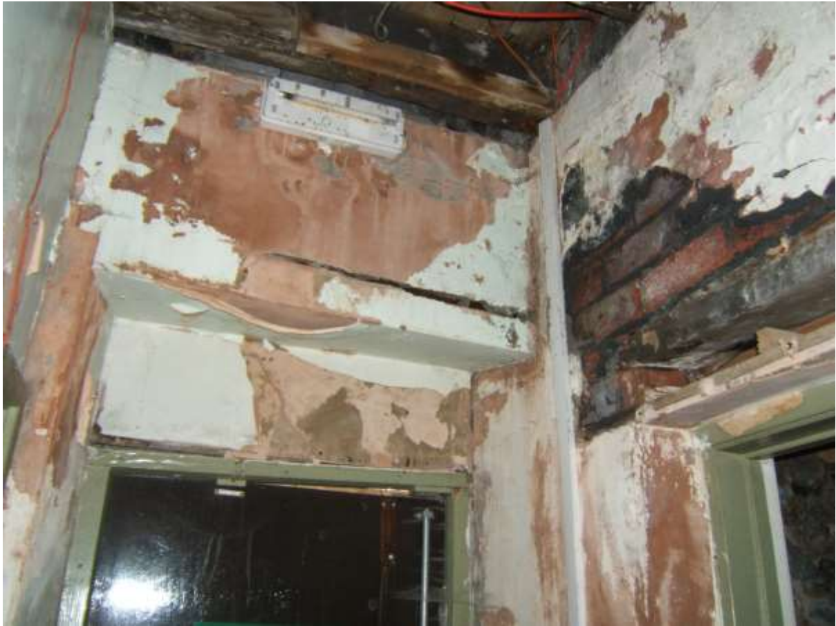
WATER DAMAGE INTERNALLY AT FIRE ESCAPE DOORWAY ON NORTH SIDE
