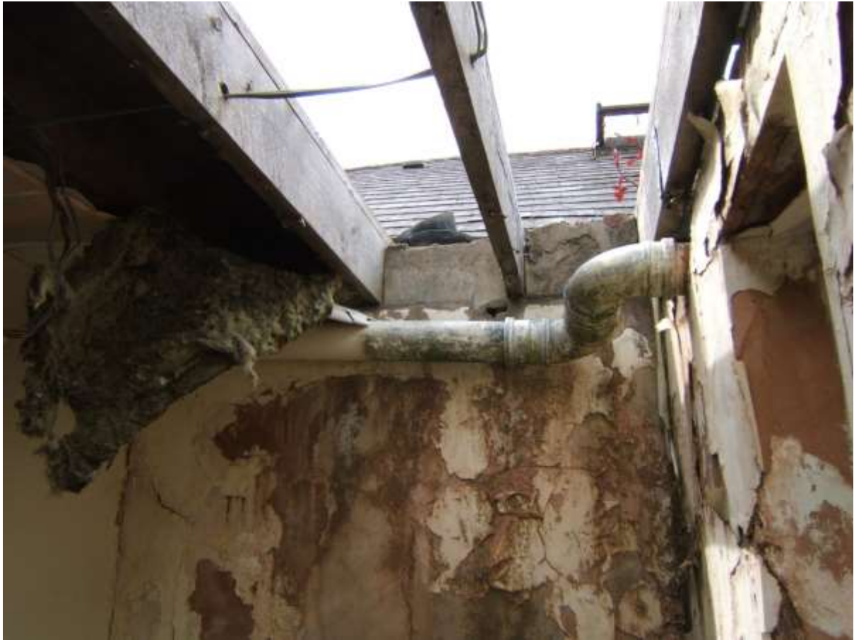
VIEW THROUGH VOID AT MISSING ROOF MEMBRANE & WATER DAMAGED WALLS
