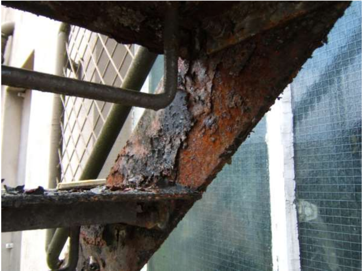
TYPICAL DEFECT ON METAL ESCAPE STAIRWAY & PLATFORMS
