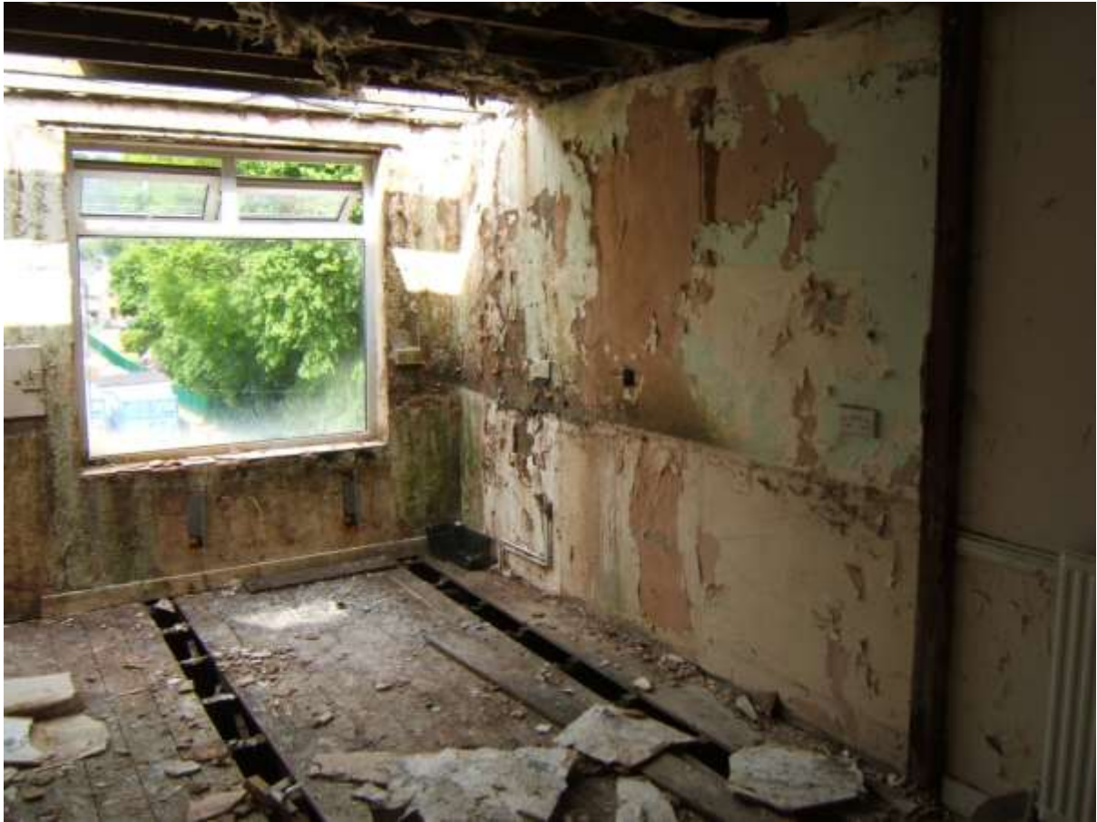
WATER DAMAGE INTERNALLY ON TOP FLOOR REAR ROOM UNDER MISSING ROOF AREA
