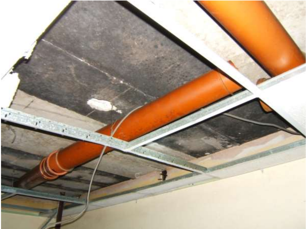
DISPLACED FOUL PIPE IN CEILING VOID OF BASEMENT
