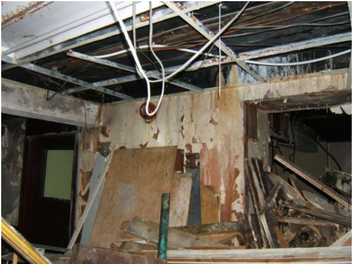
GENERAL VIEW THROUGH REAR BASEMENT ROOM SHOWING DETERIORATION INTERNALLY FROM WATER PENETRATION FROM ABOVE
