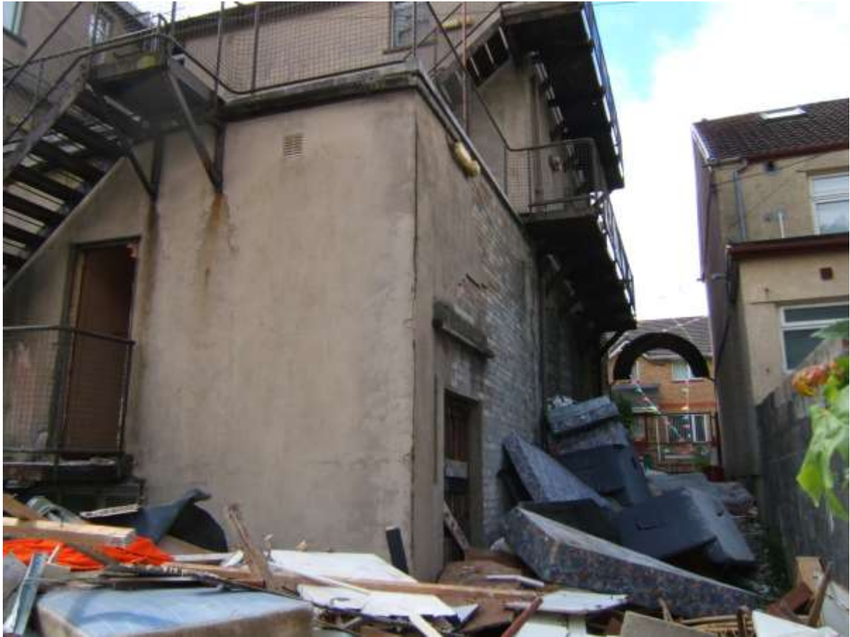
REAR NORTH EAST CORNER WITH RENDER DEFECTS TO BOTH WALLS
