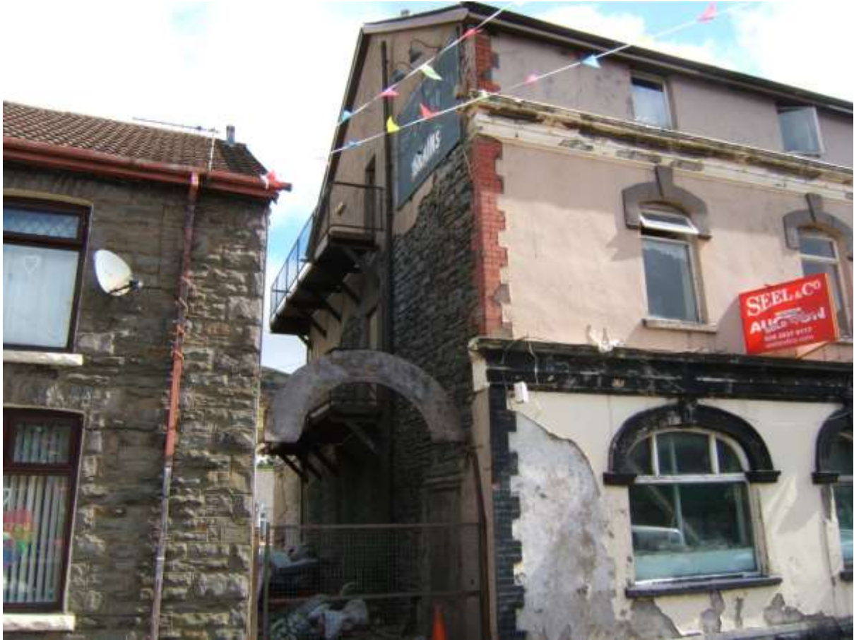
SIDE GABLE WALL SHOWING DEFECTIVE RENDER
