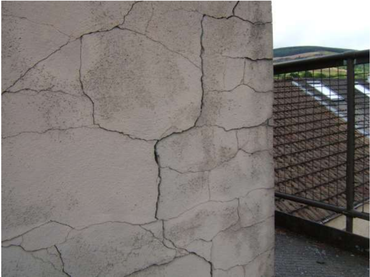
RENDER FAILURE AT REAR UPPER NORTH EAST CORNER
