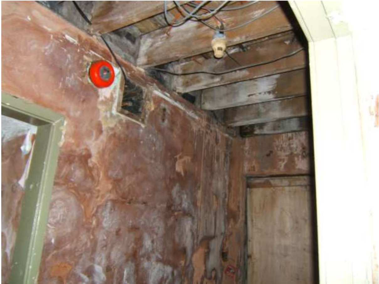
WATER DAMAGED REAR WALL & FLOOR JOISTS IN REAR
