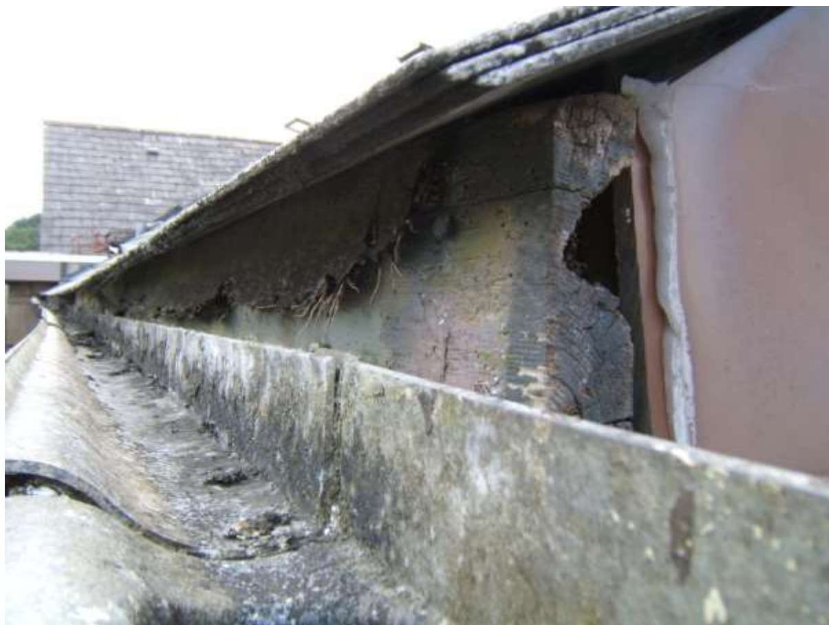
TIMBER FASCIA AT REAR UPPER MAIN ROOF EDGE WITH WOODWORM & ROT
