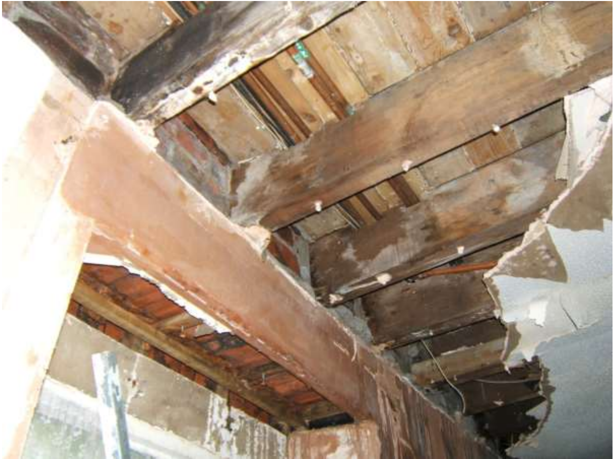
WATER STAINED TIMBER FLOOR JOISTS WHERE BUILT-IN TO REAR WALL ON UPPER FLOOR
