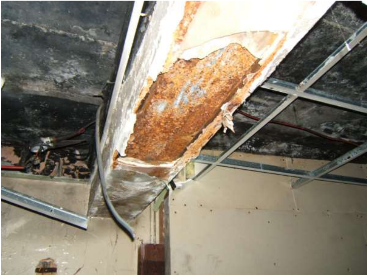
SURFACE RUST ON STEEL SUPPORTING MEMBER IN REAR BASEMENT AREA
