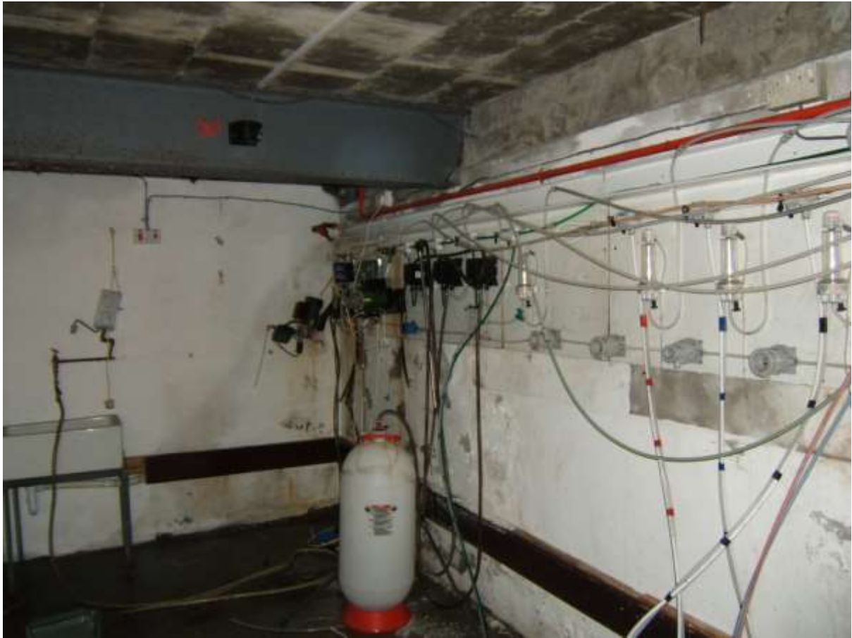
FRONT INTERNAL ROOM IN BASEMENT WITH WATER INGRESS FROM LEAKING WATER PIPE
