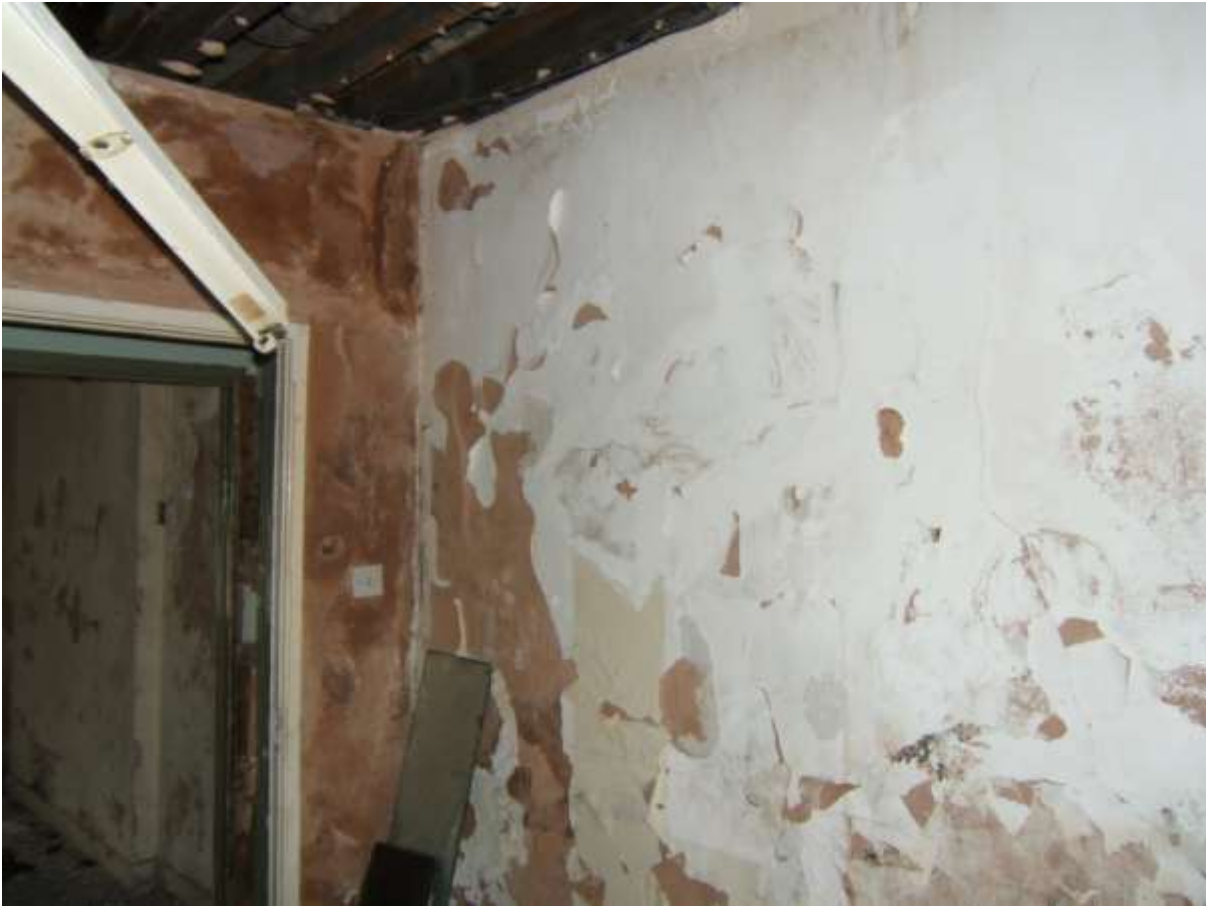
PLASTER DAMAGED GABLE WALL ON NORTH SIDE FROM WATER PENETRATION
