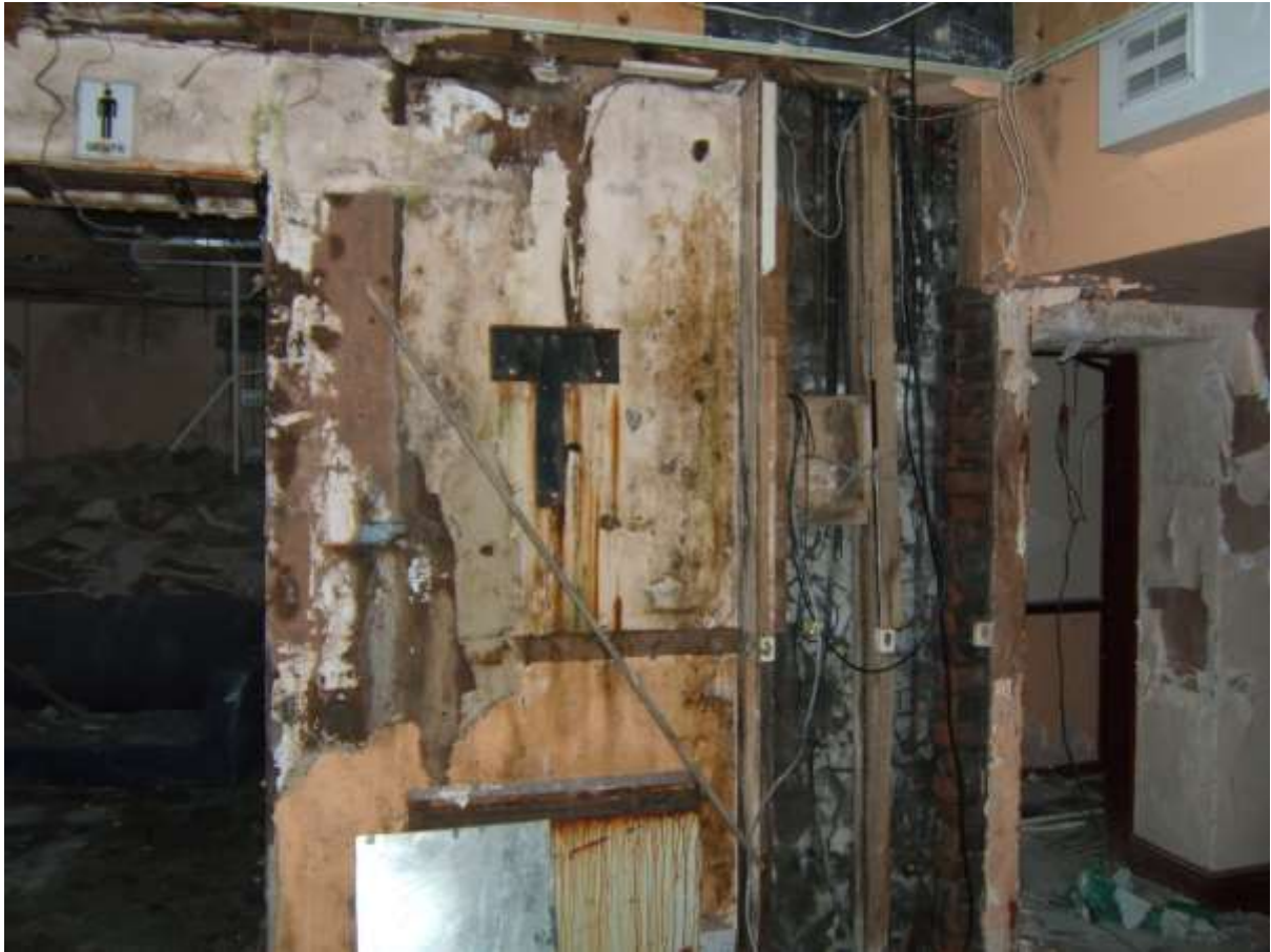
WATER DAMAGED INTERNAL WALL IN FORMER BAR AREA
