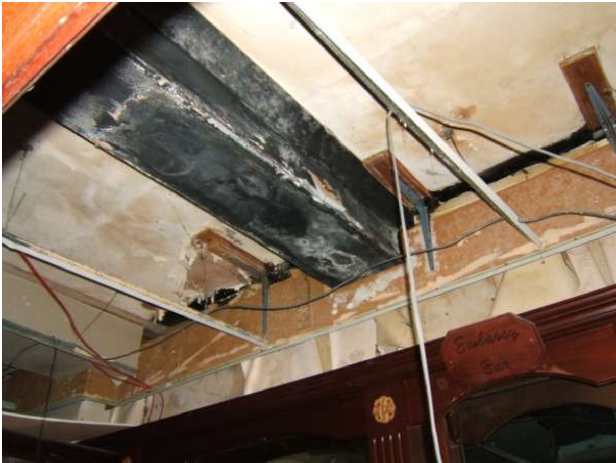
BOXED-IN STEEL SUPPORTING MEMBER IN FORMER BAR AREA ALONGSIDE NORTH GABLE WALL WITH WATER DAMAGE
