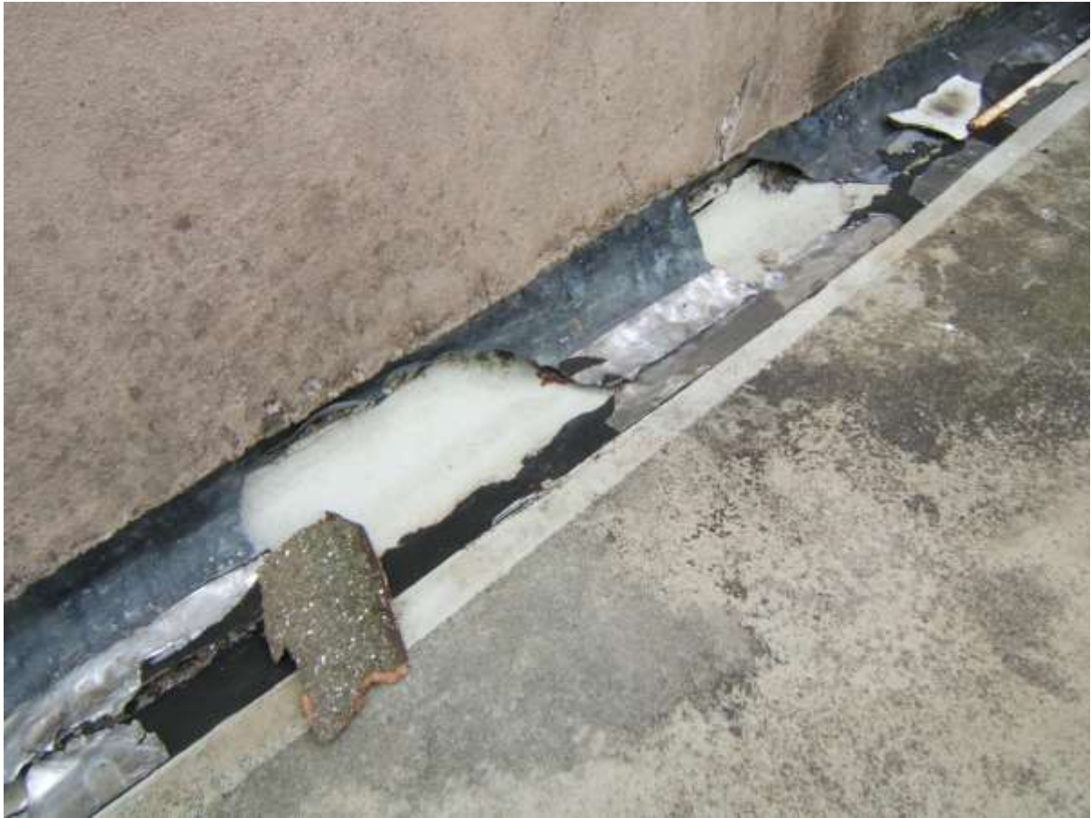
MISSING LEAD FLASHING AT LOWER FLAT ROOF JUNCTION WITH WALL
