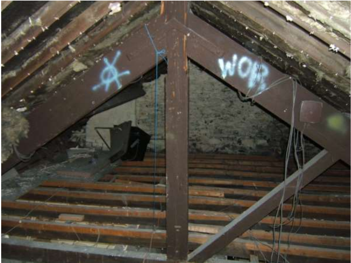
PRINCIPLE TIMBER TRUSS WITH MISSING DIAGONAL SUPPORT STRUT IN ROOF VOID
