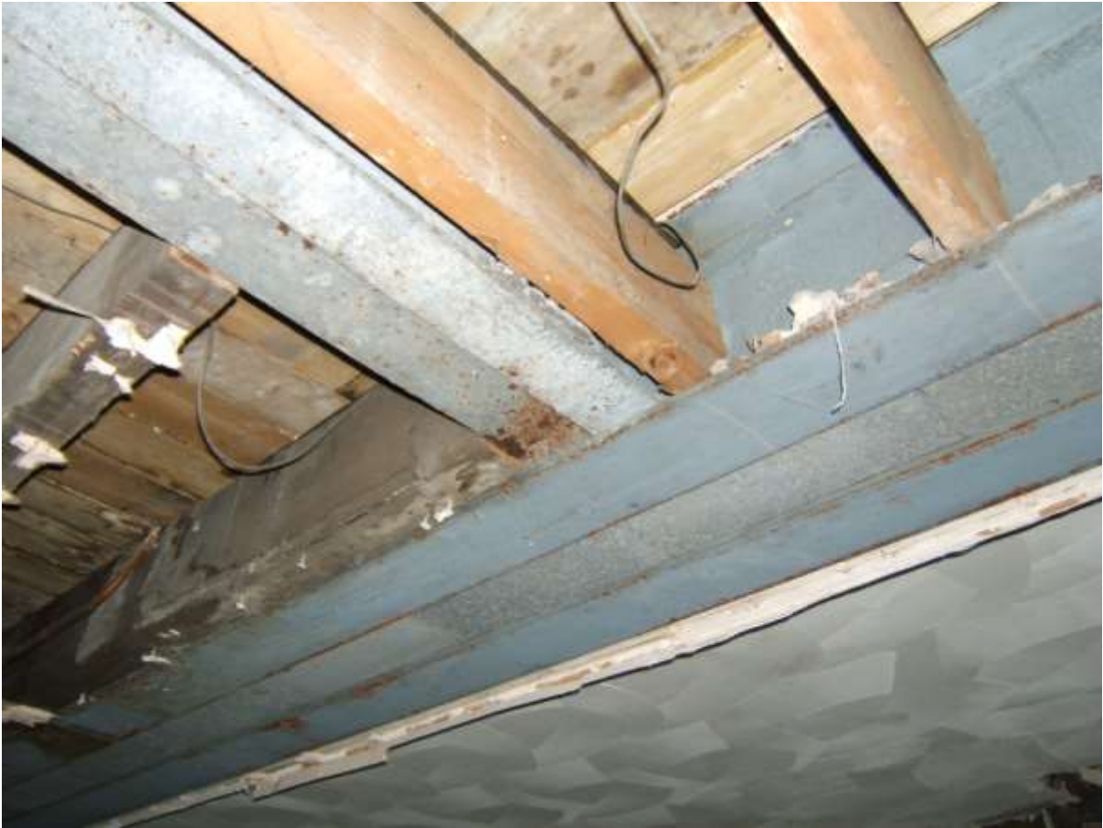
STEEL SUPPORTING MEMBERS ON UPPER FLOOR WITH SURFACE RUST
